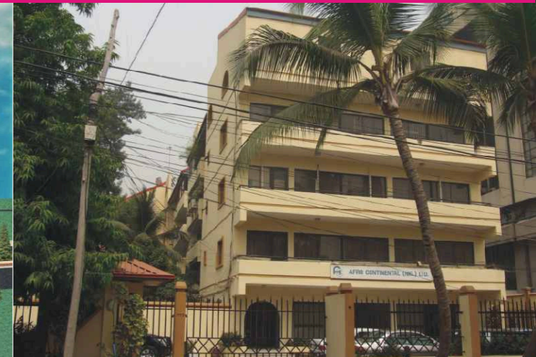
Residential Development, Ikoyi, Lagos
