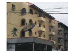
Residential Development, Ikoyi, Lagos
