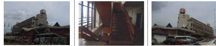
UAC BUILDING BUILDING TYPE: OFFICES BLOCK DEVELOPMENT LOCATION: ABUJA CLIENT: UAC
