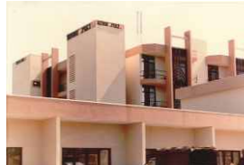
Office block for CAPL, Lagos
