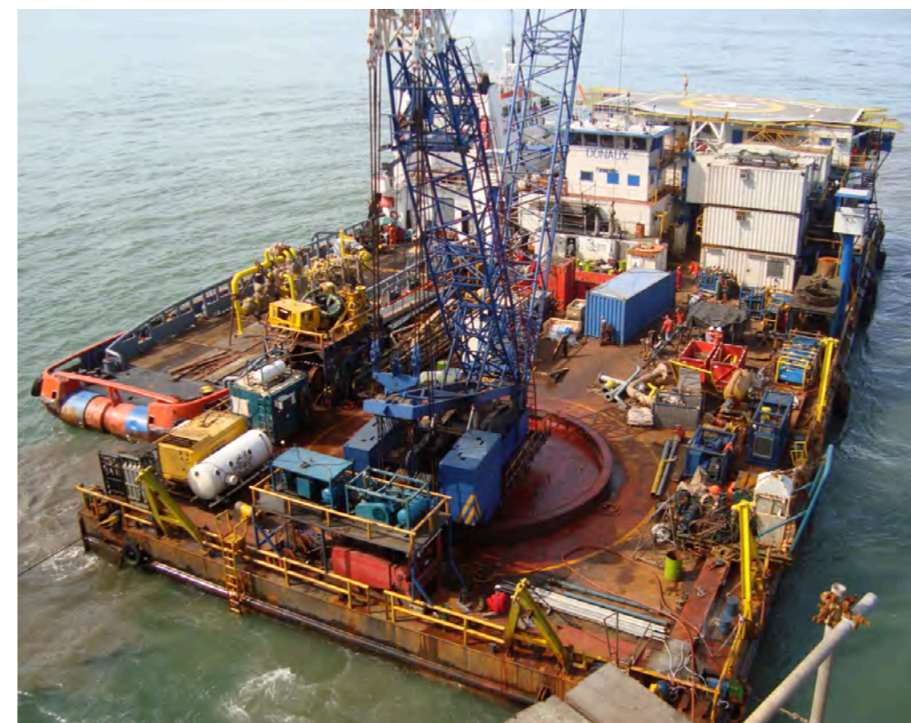
Photograph predates installation of the pipelay system on the Barge
